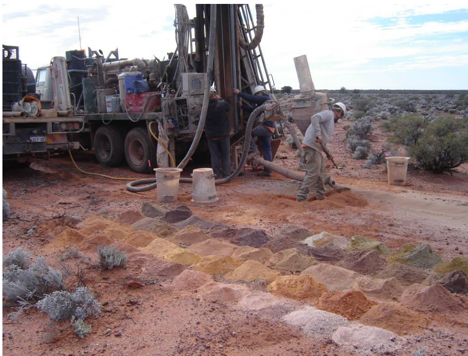
Photo 1. Air-core Drilling, Monsoon Prospect near Challenger gold mine, South Australia.
