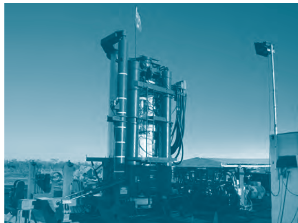
Raise Bore – Drilling Ventilation Shaft Pilot Hole
