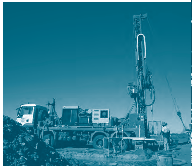
Challenger Surface Drilling
